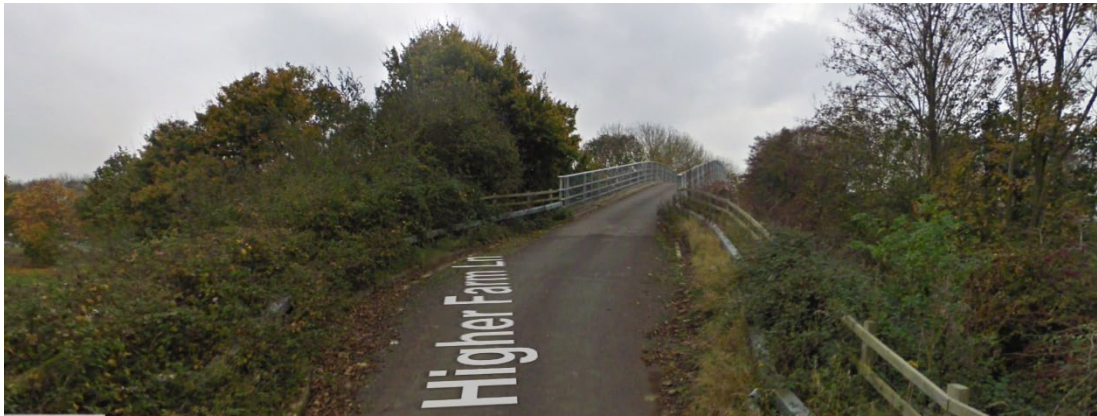
Figure 4: Higher Farm Overbridge from north side approach 42
